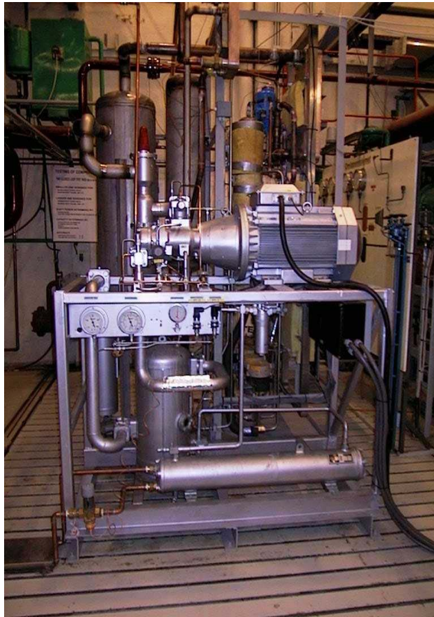
Figure 6: Laboratory plant during erection. Liquefaction capacity 1 tonne LNG/day; Photo: SINTEF
